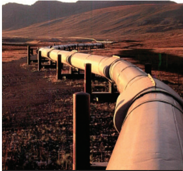
Trans-Sahara Gas Pipeline
