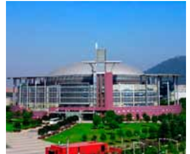
China Electronics Technology Group Corporation's 38th Research Institute in Its New Facilities
