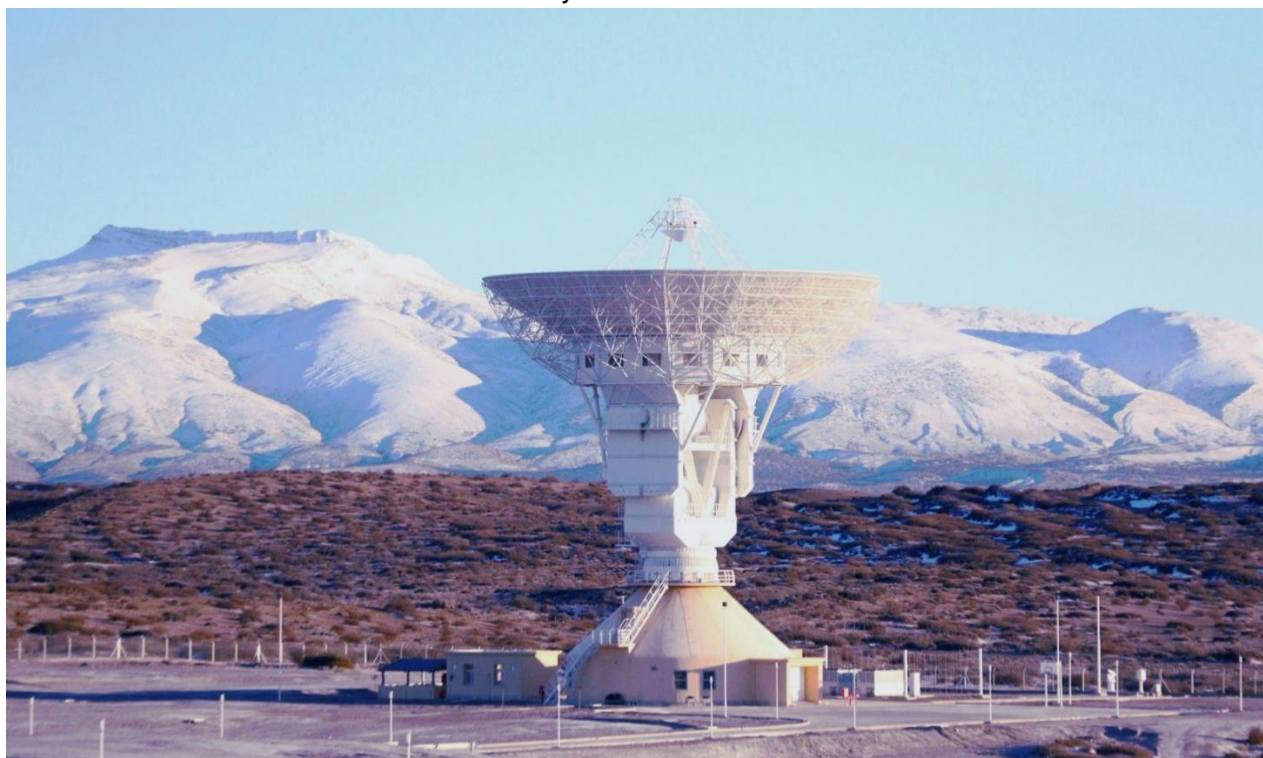
The Espacio Lejano Station in Neuquén Province, Argentina. (Source: Wikipedia)
