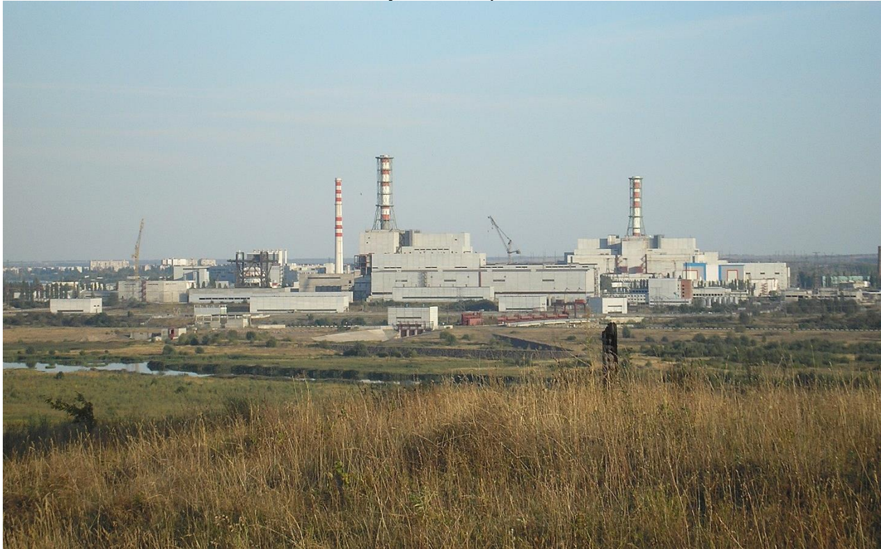
Kursk nuclear power plant. (Source: Wikipedia )
