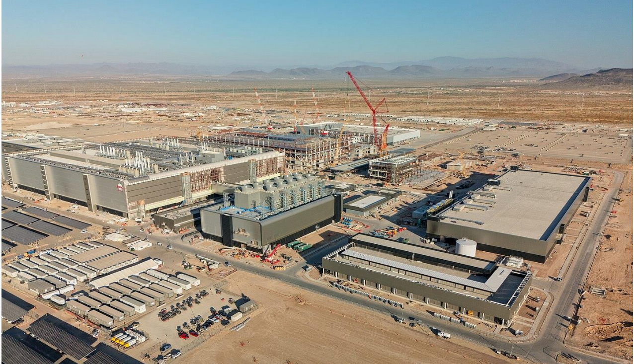
TSMC's Fab 21 under construction in Phoenix, Arizona in November 2023. (Source: Wikipedia )
