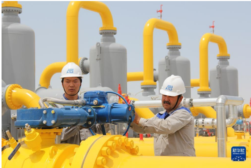
Workers operate on a station of the China–Central Asia Natural Gas Pipeline. (Source: Xinhua)
